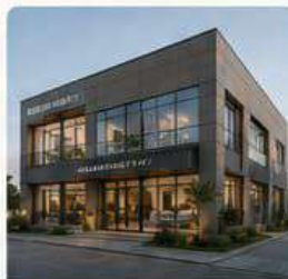
COMMERCIAL COMPLEX by Sri Builders Coimbatore
